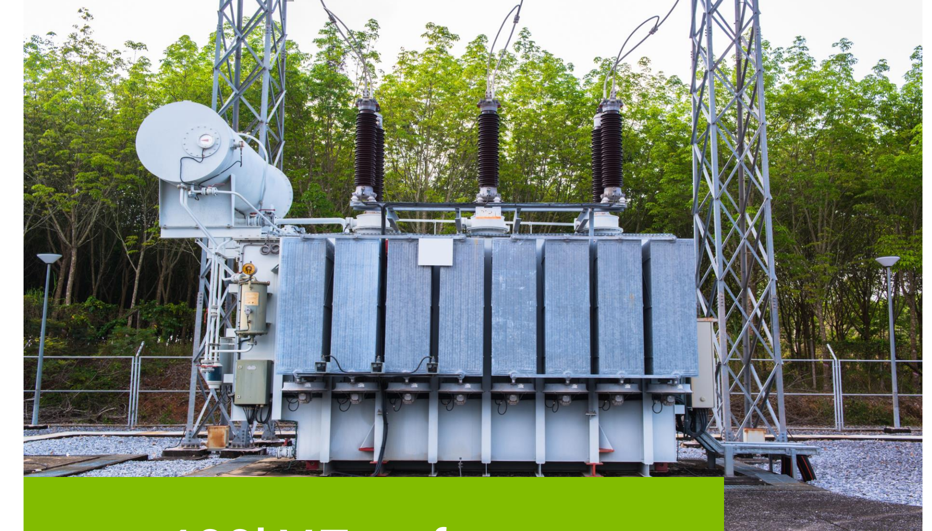
132kV Transformer
